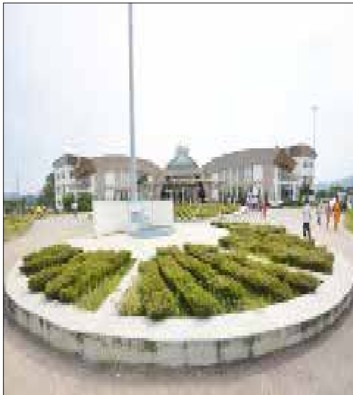
GNRC Hospital, North Guwahati
